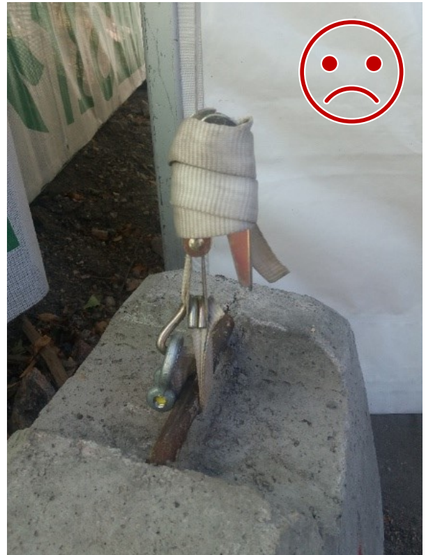
Figure 6 WRONG. The hook is not locked, should be locked with a shackle to the fixing point.
