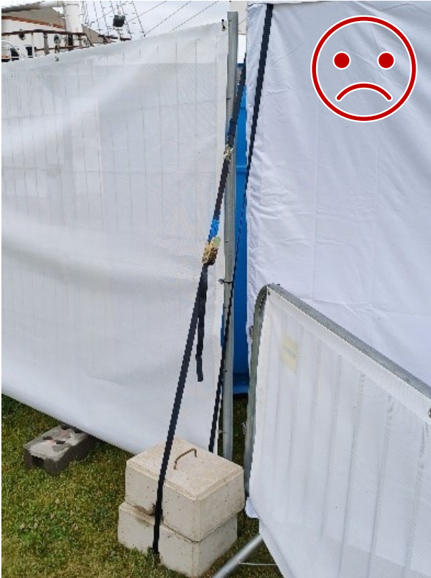
Figure 11 WRONG . The weights are not locked to the strap or to each other. The stack will fall, and the strap will not hold as the structure shifts.
