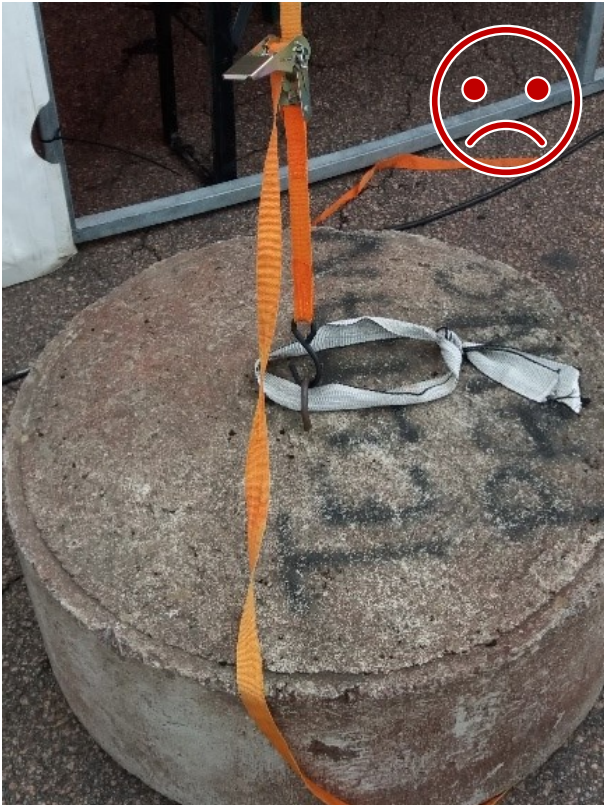
Figure 7 WRONG. The S-hook is not lockable. The hook will come loose as the structure shifts.
