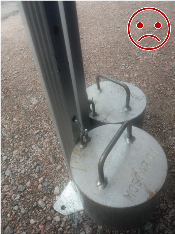
Figure 9 WRONG . The steel hook does not lock into the structure, and the steel will cut the aluminium as lift shakes the tent.
